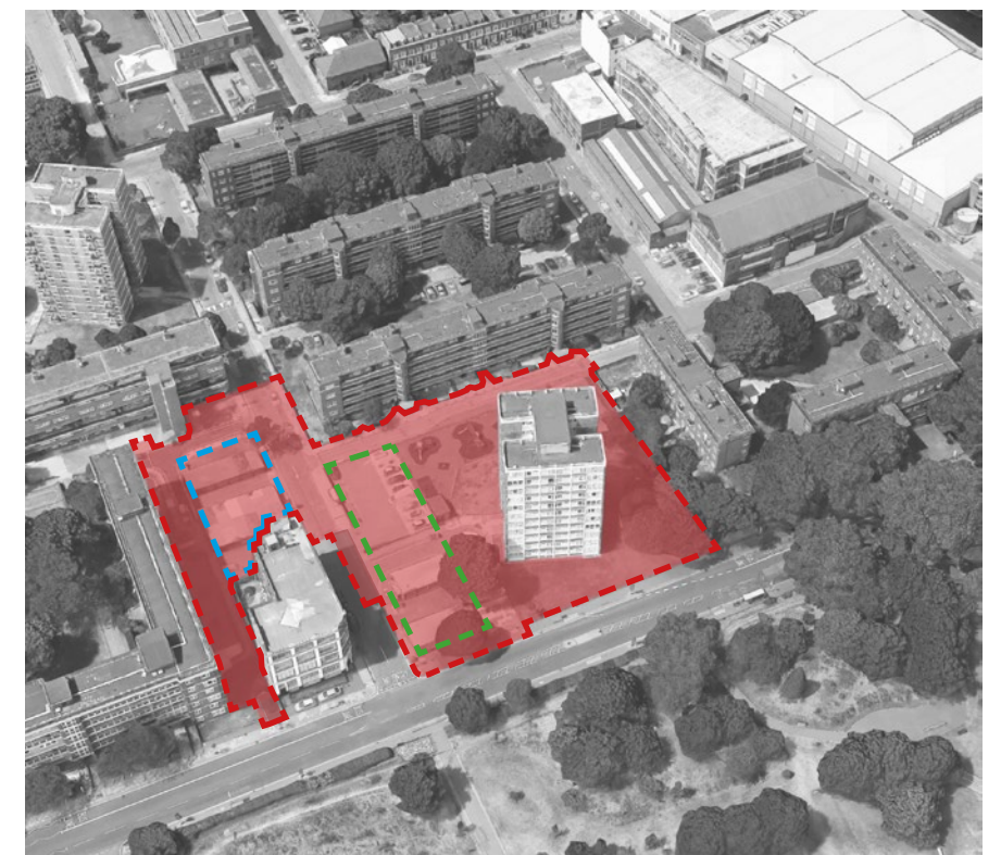
4. Aerial view looking West
