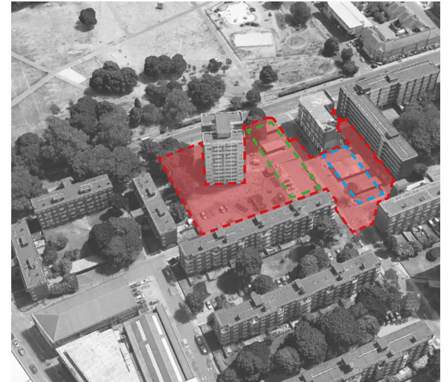
2. Aerial view looking East
